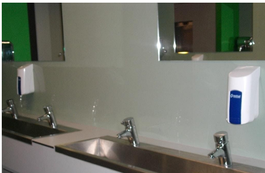
Between the girls and boys toilets are shared sinks
